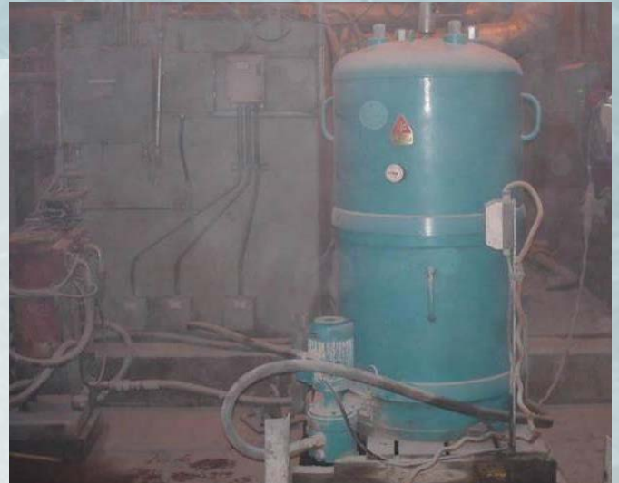
CJC™ Fine Filter HDU 427/108 installed at BHP Minera Escondida
