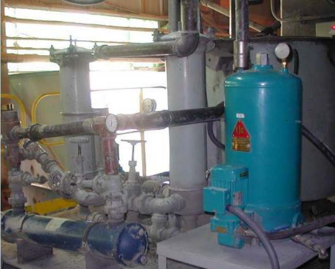
A CJC™ Fine Filter installed on Crusher 4 at Codelco Mine site in Chile
